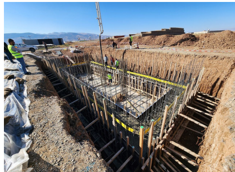
■ Reinforced concrete substructure works
