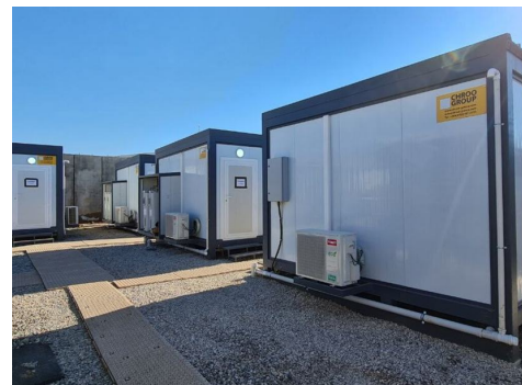
■ Finished containerized units on site
