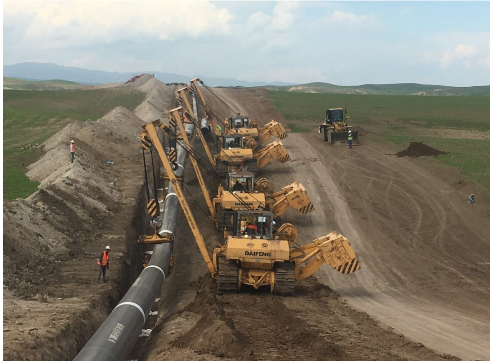
■ Pipeline construction fleet, Kurdistan Region
