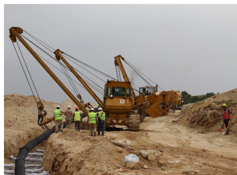
■ Trench works and bedding
