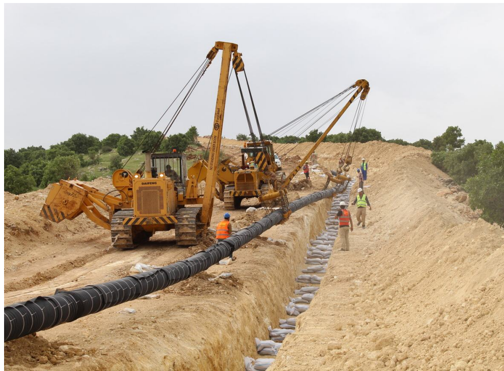
■ Pipeline lowering in with sidebooms, Kurdistan Region
