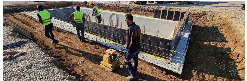
■ HSE managed foundation works, certified equipment and trained crews
