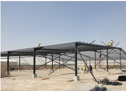
■ Steel frame erection, Erbil
