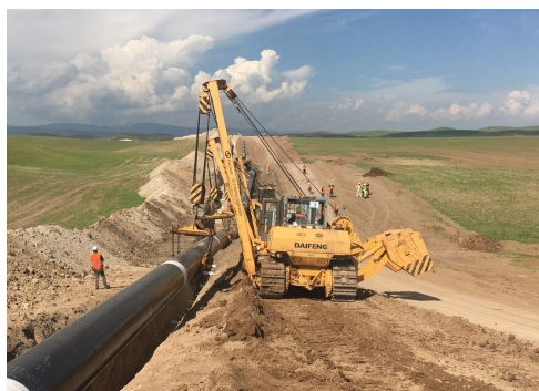
■ Right of way and stringing
