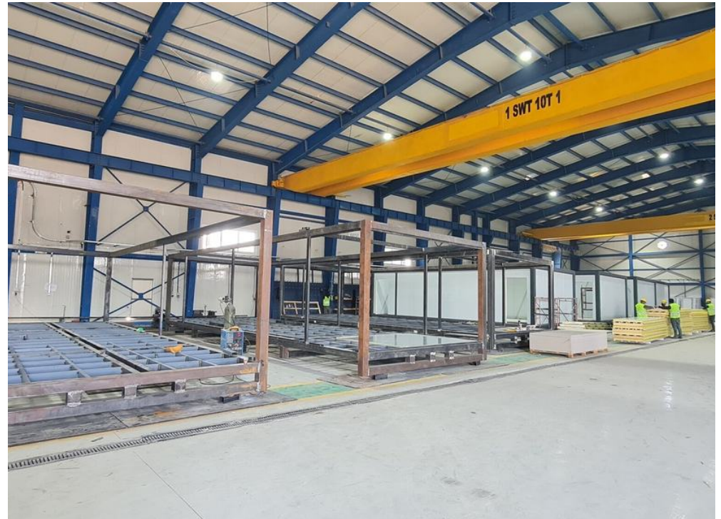
■ Chroo fabrication workshop, containerized unit production
