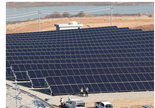
■ Utility scale solar plant under construction
