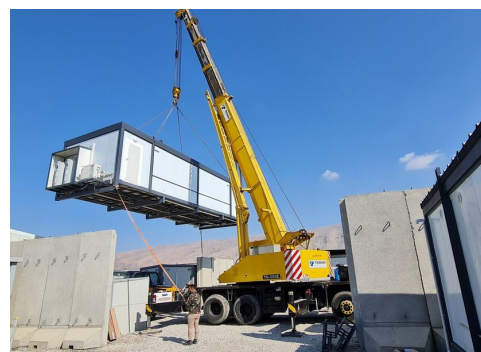
■ Camp unit installation by crane
